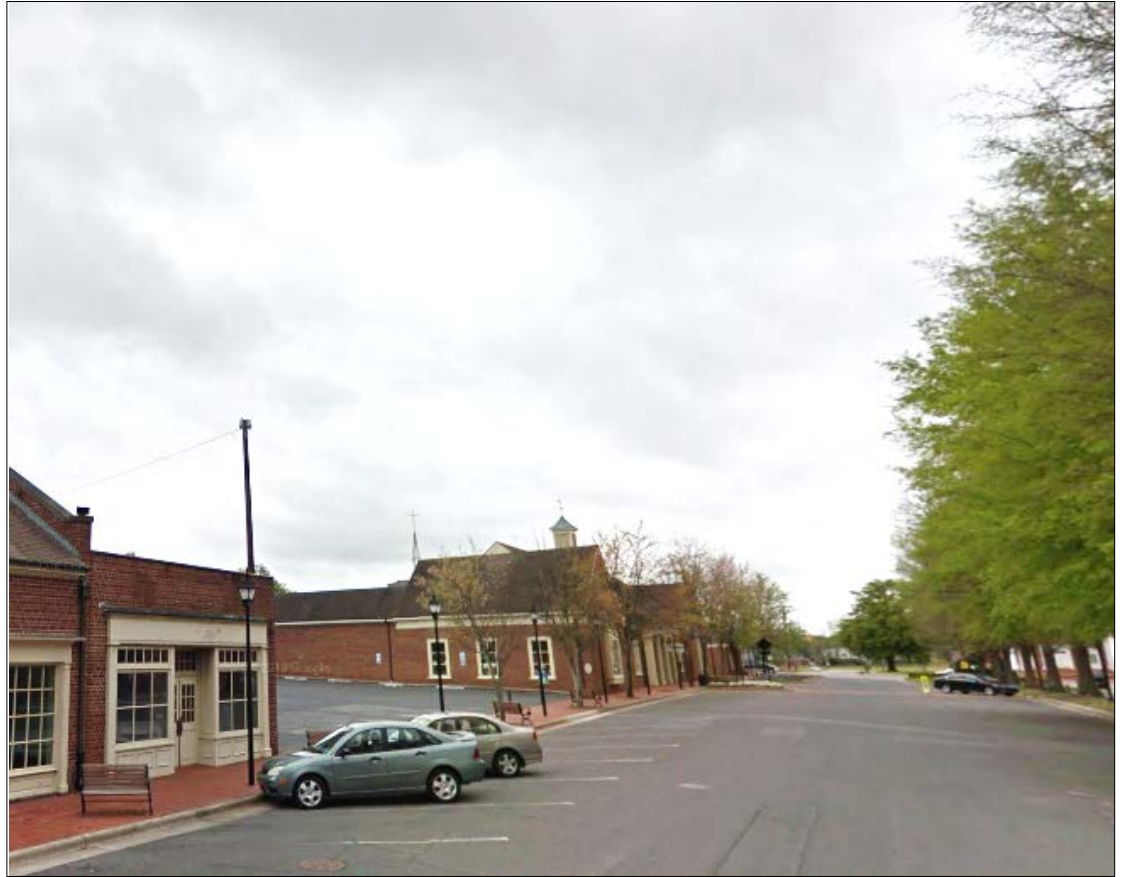
Existing view of West Avenue looking south from center block
